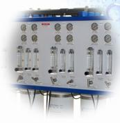
Pure Aqua's needle valve flow meters installed on panel for regulation of flow on electrodeionization system.
